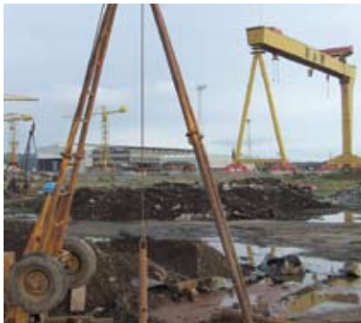
Borehole drilling
