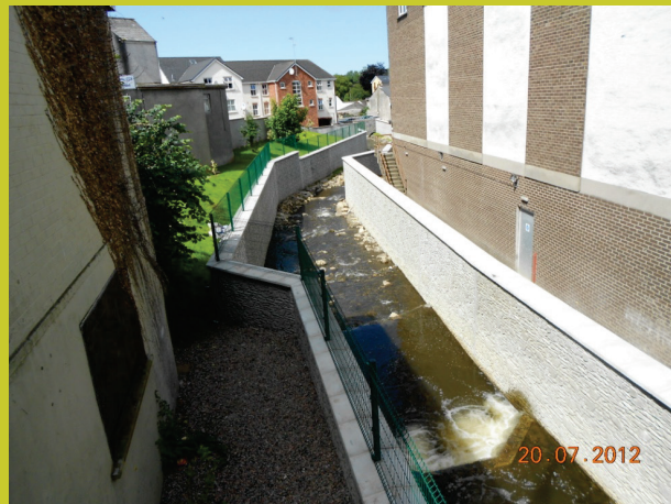
After scheme was completed
