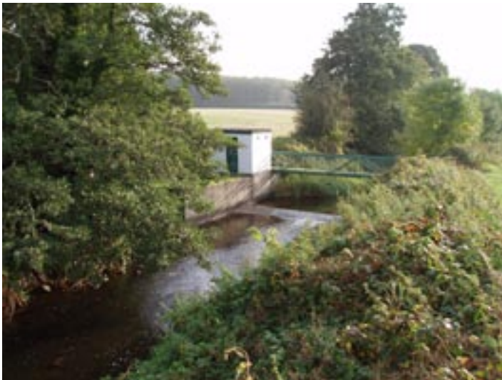
River flow gauging station (Courtesy of Rivers Agency)
