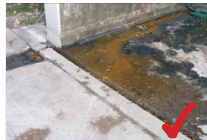
Silage clamp with well maintained channels draining to effluent tank.
