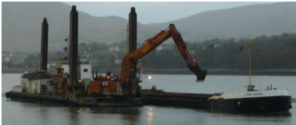
Figure B2 Typical Backhoe and Barge Combination
