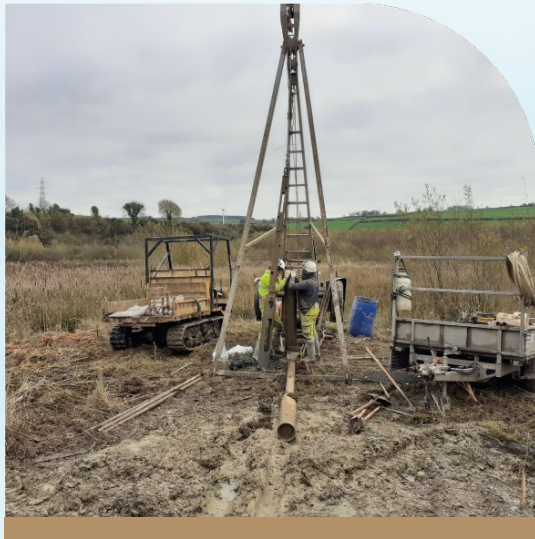
Drilling of Borehole – Nov 21
