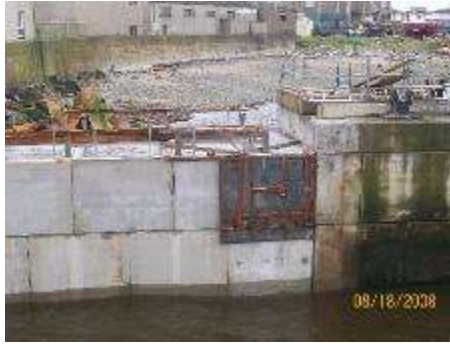
Figure 5 – Example of in situ concrete formwork from Kilkeel
