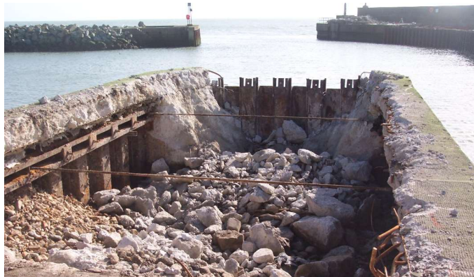
Figure 1 – Example of slab demolition at Kilkeel Harbour
