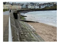
(2) Part demolition (east of the culvert only) of the existing noncompliant pedestrian access ramp (with regards gradient and low level spur) and construction of a new, compliant, <u>pedestrian</u> <u>access ramp with stepped</u> <u>access for ambulant persons.</u> The new ramp shall comply with BS 8300 *Design of an accessible and inclusive built environment*, and
