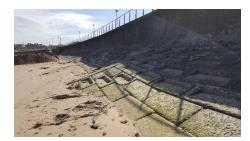
(3) <u>Remedial works to 150m of</u> <u>existing revetment</u> (the total length of existing revetment is 1000m): Replacement of the damaged precast revetment units in the revetment and new sheet pile scour protection seaward of the existing sheet piles which have deteriorated beyond their useful life.
