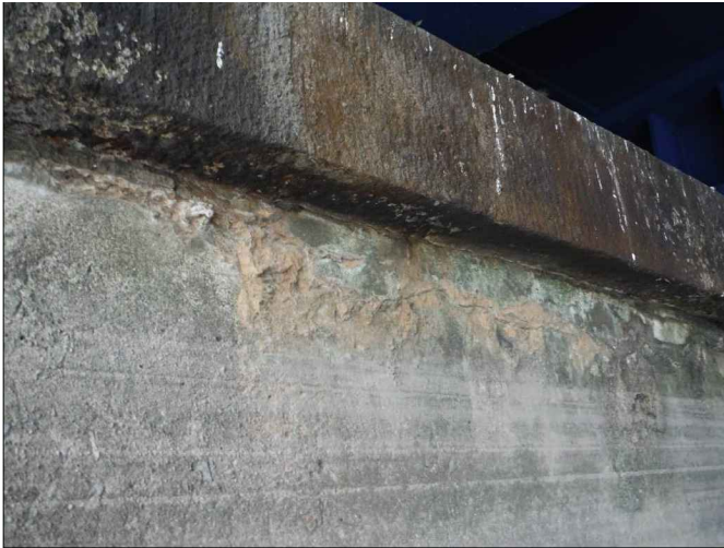
Photo 1 - Pier 2 Horizontal crack
