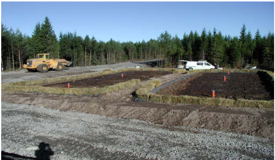
Fig.7. Full scale treatment filters showing surface spray irrigation and construction
