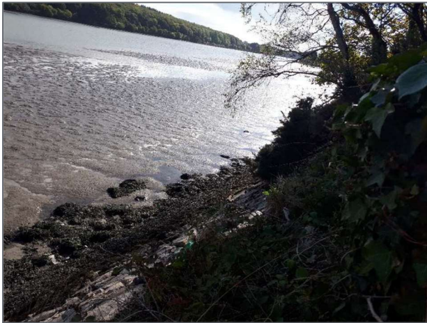
Plate 4: Mudflats – Temporary Working Platform to be Placed on Top of Mudflats with Geogrid Separator Layer
