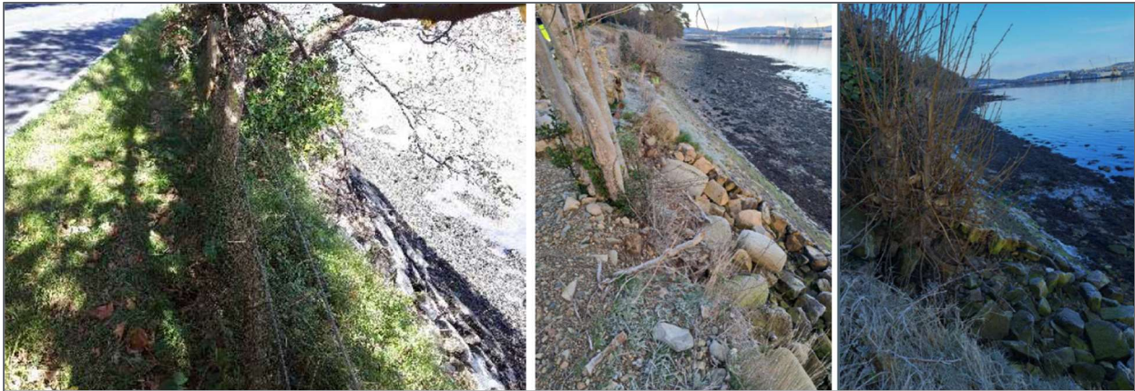
Plate 3: Existing Rock Armour Section
