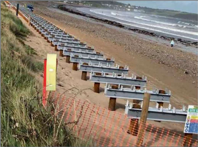
Plate 5: Examples of Piled Boardwalk
