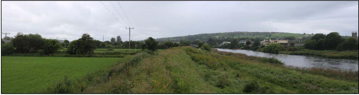
Figure 14-8: On bank of River Foyle, off site
