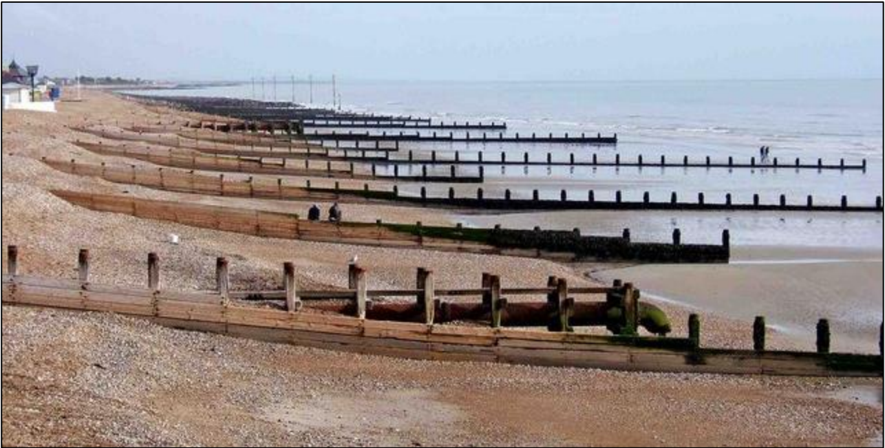
Figure 3.7: Example of wooden groynes at Bognor Regis
