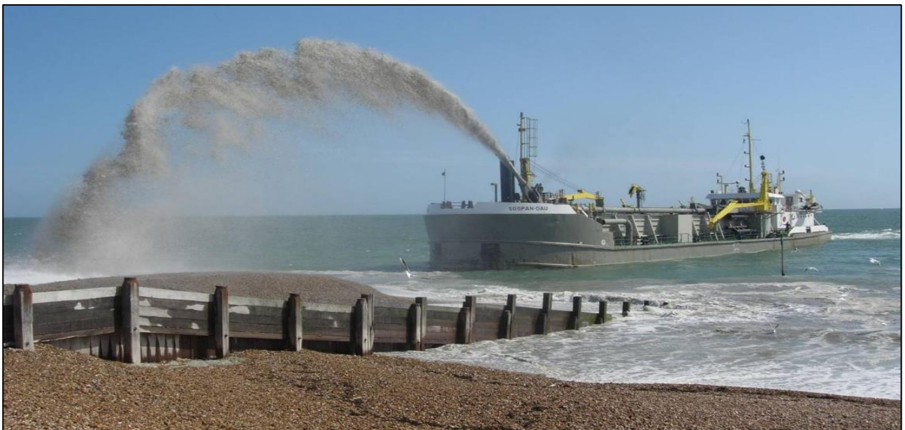
Figure 3.13: Beach nourishment material being placed onshore using a rainbow spray technique
