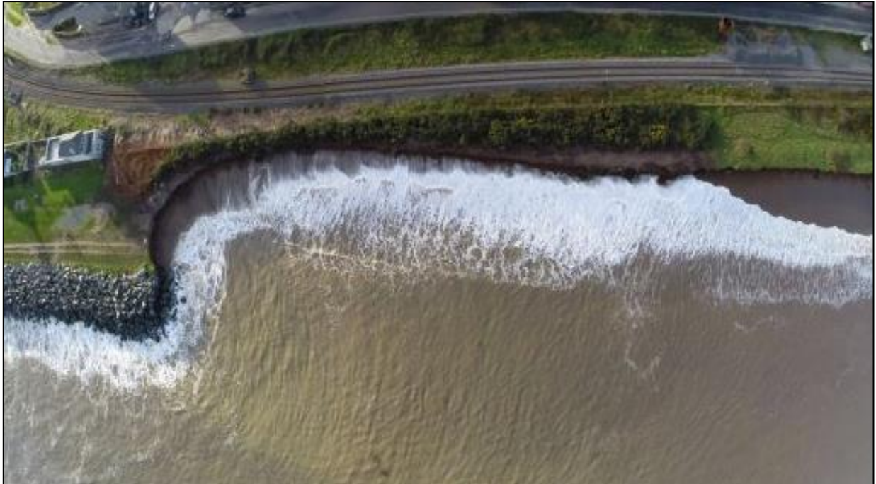
Figure 3.5: Example of terminal erosion at the Murroughs, Wicklow (c.2014)
