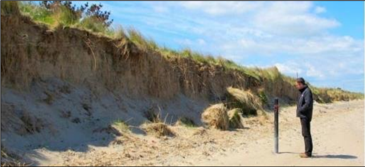
Figure 3.15: Example of over-steepened and unstable dune face at Portrane, Fingal.
