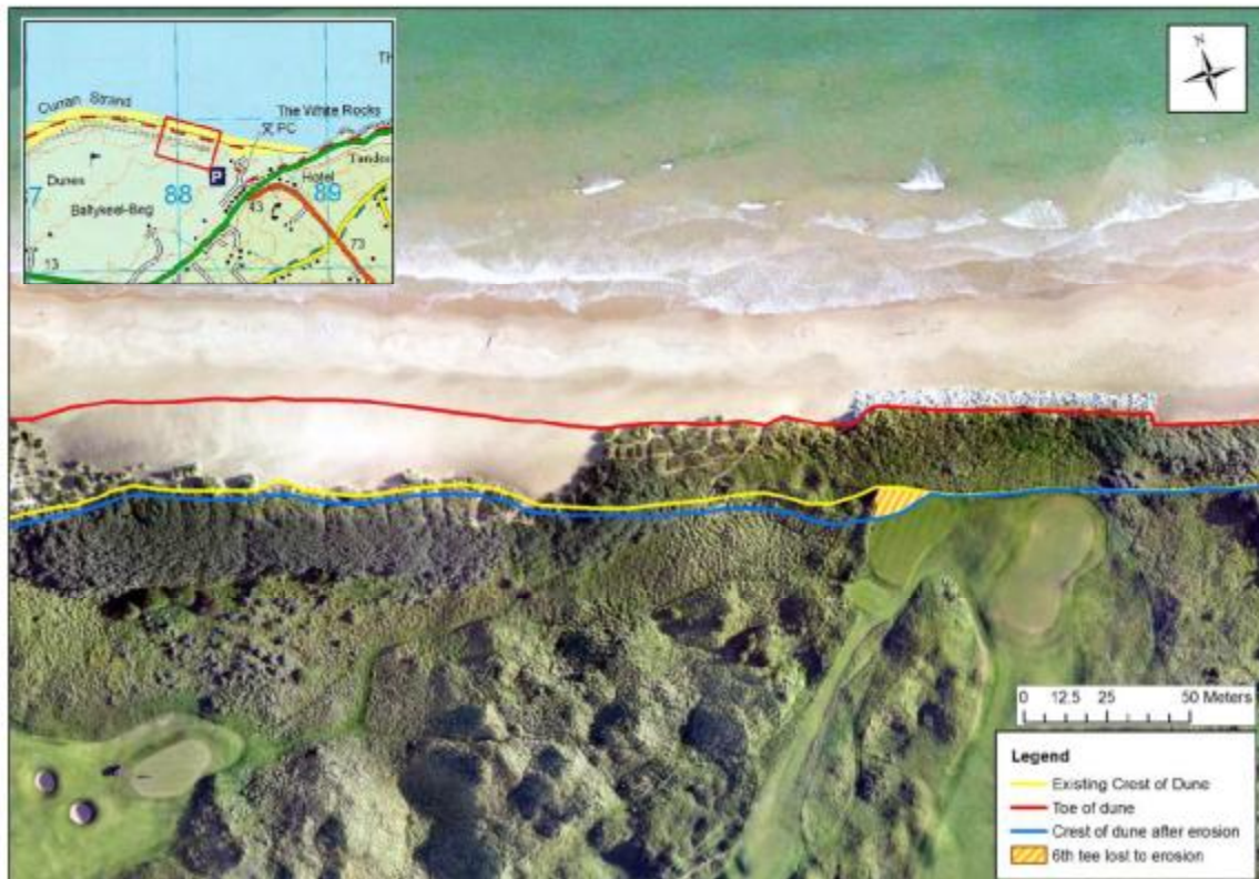
Figure 3: Area of hinterland that could be lost to coastal erosion under 1 in 100 year event from NW with existing rock revetment and gabions in place (RPS, 2017).
