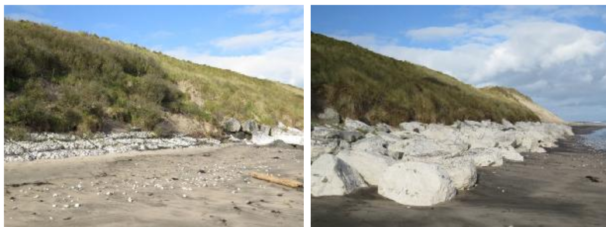
Figure 2: Existing gabions and rock revetment
