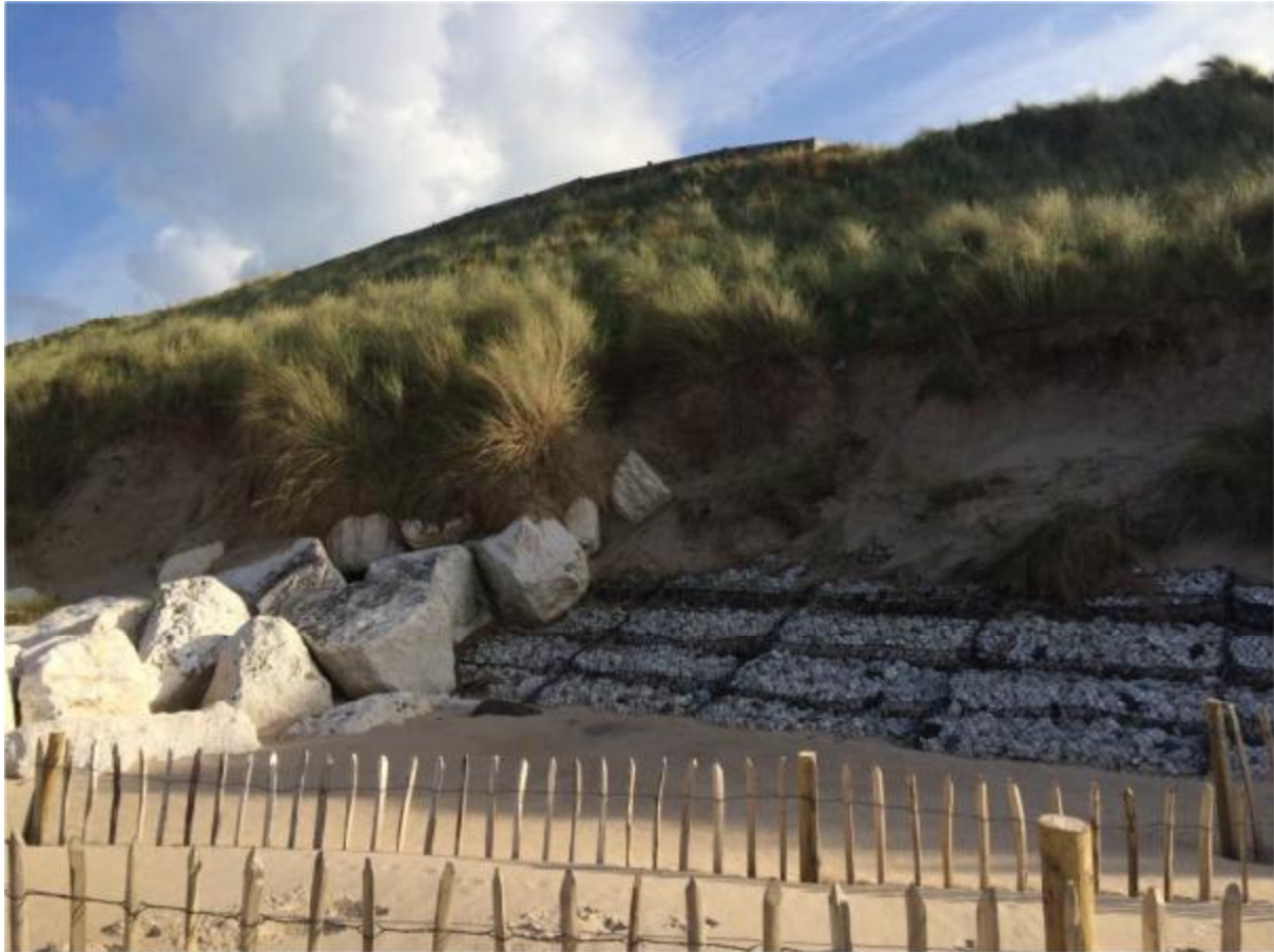
Figure 4: Previous sand trap fencing to eastern end of existing rock revetment.
