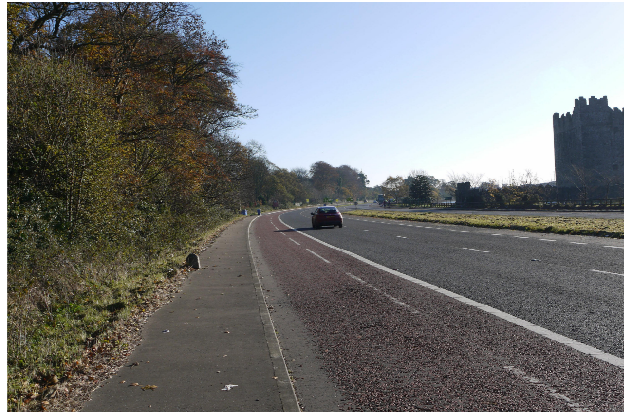
VIEW OF BRIDGE AND ADVANCED SIGNAGE (VMS ON) FROM A2 APPROCH TO ROUNABOUT (FROM NEWRY SIDE) PHOTOMONTAGE NO.8
